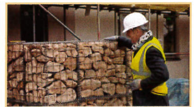
The delivery and usage of Smiths' gabion stone
